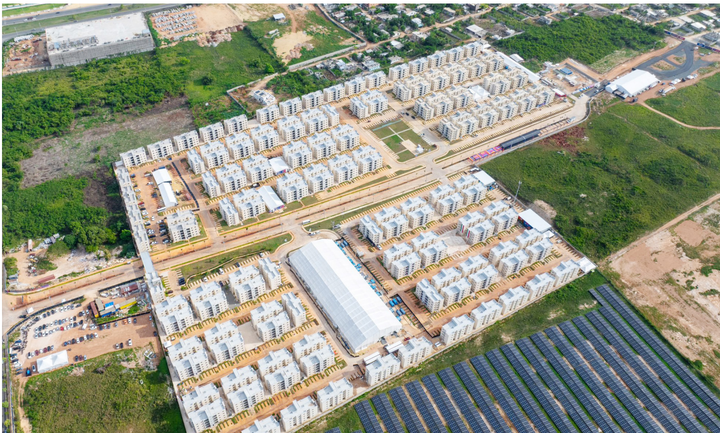
Aerial view of the residential complex that will house more than six thousand athletes participating in the XXV Central American and Caribbean Games.
