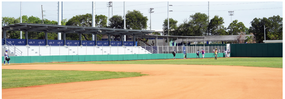
A view of the renovated Baseball Stadium #3, located at the Olympic Center.
