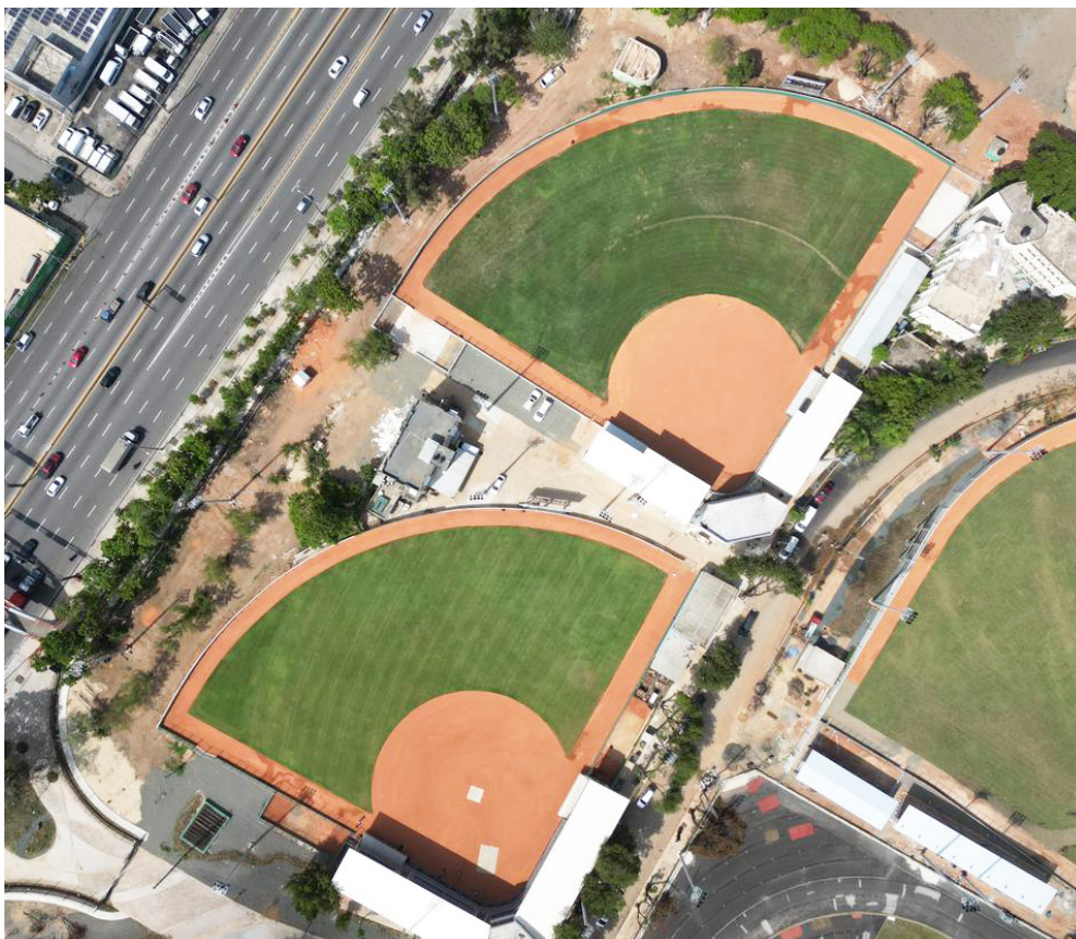
Softball B Stadium now boasts new bleachers, locker rooms, a drainage system, and LED lighting.
