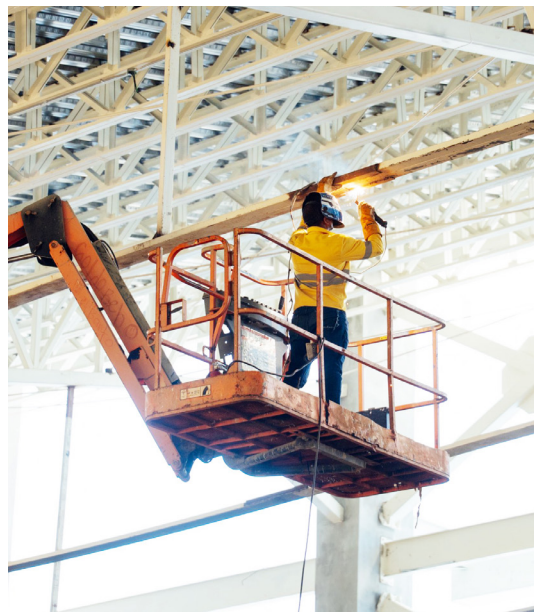
A worker is working in the Combat Pavilion.
