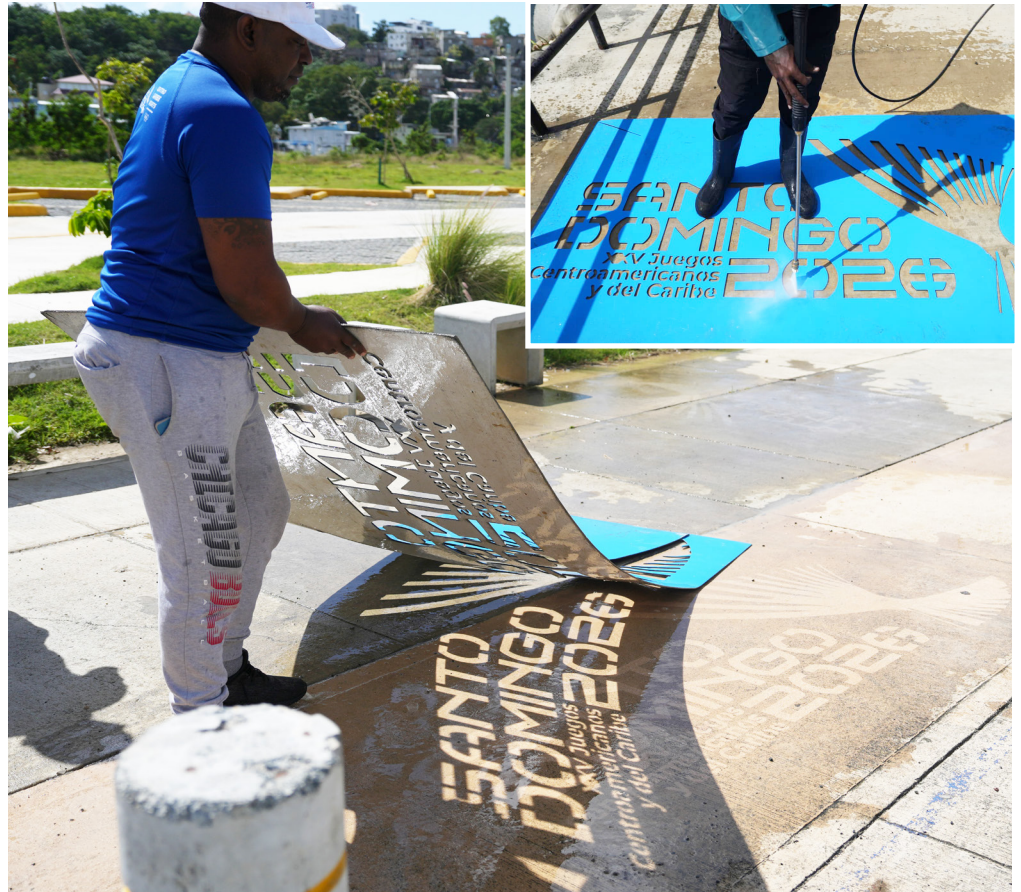
The reverse “graffiti” process consists of cleaning part of the sidewalk with pressurized water.
