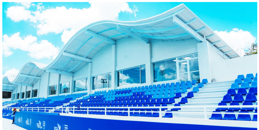
Aquatic Center: structural improvements and general facility upgrades.
